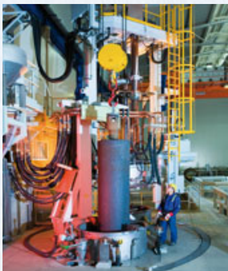
Special Steel Plant Extension
